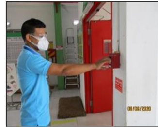
External photo(s) of the production unit(s) Fire alarm check.JPG
